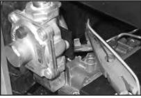
Figure 33: Spill Switch Wires **Connect to Thermocouple.**
